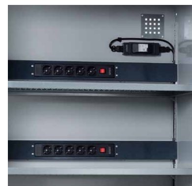
Rear panel installation
