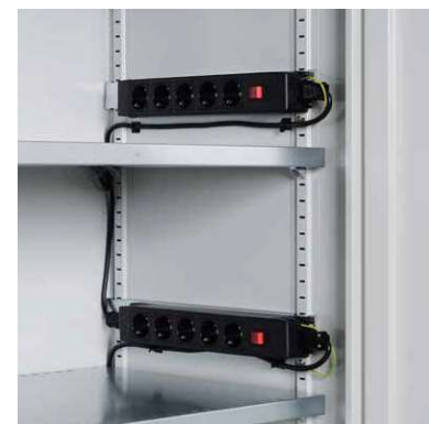
Side panel installation
