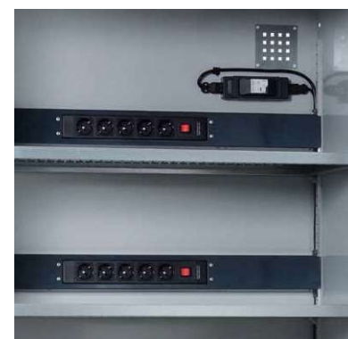
Rear panel installation
